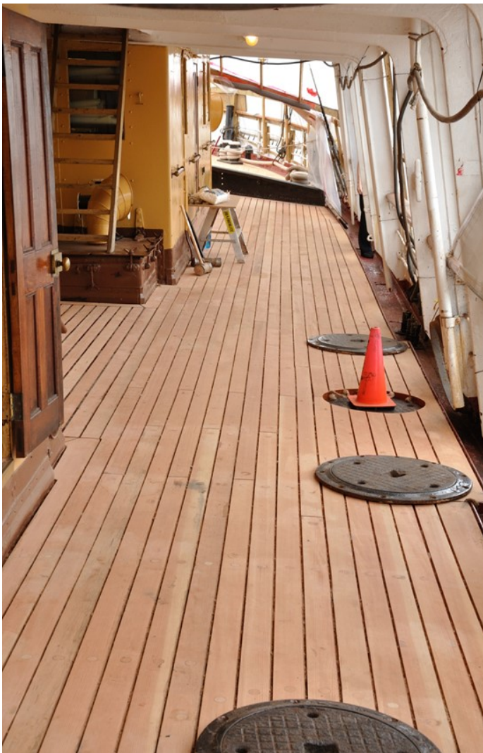
New decking almost complete with only the caulking left to finish. (Andy Sherin photo)
