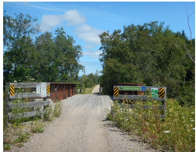
Fig 3 - An old railway bridge, well maintained by local groups.
