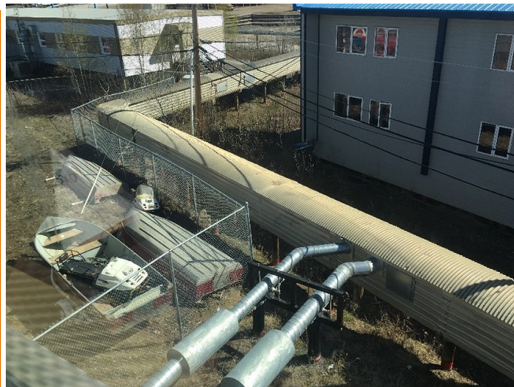
Fig.7 The utilidoor system in Inuvik provides above ground plumbing in this permafrost landscape.
