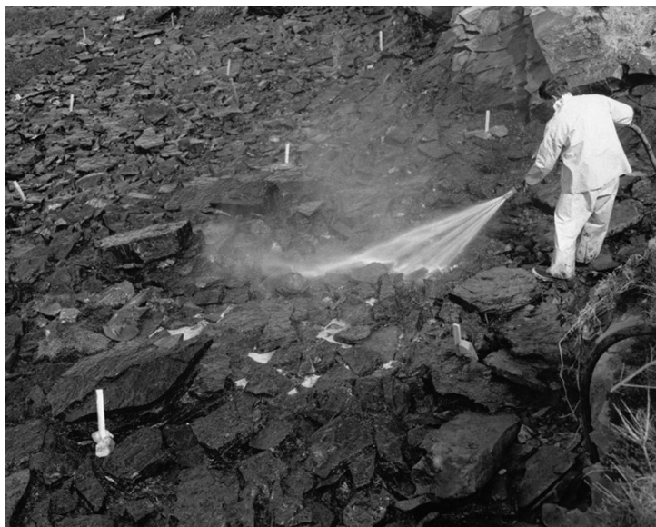
Figure 3. Steam-cleaning a rocky shoreline coated with stranded oil.
